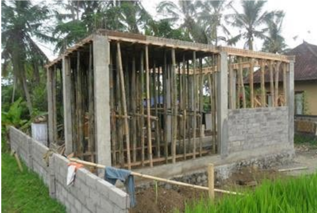
Siddharlo's Guest House under construction
